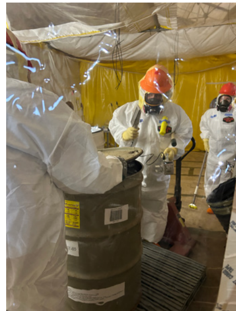
In order to ship the de-nested TRU waste, the waste needed to be removed from their storage containers and placed into certified shipping containers. Operators perform removal activities in a plastic hut, using full personal protective equipment.
